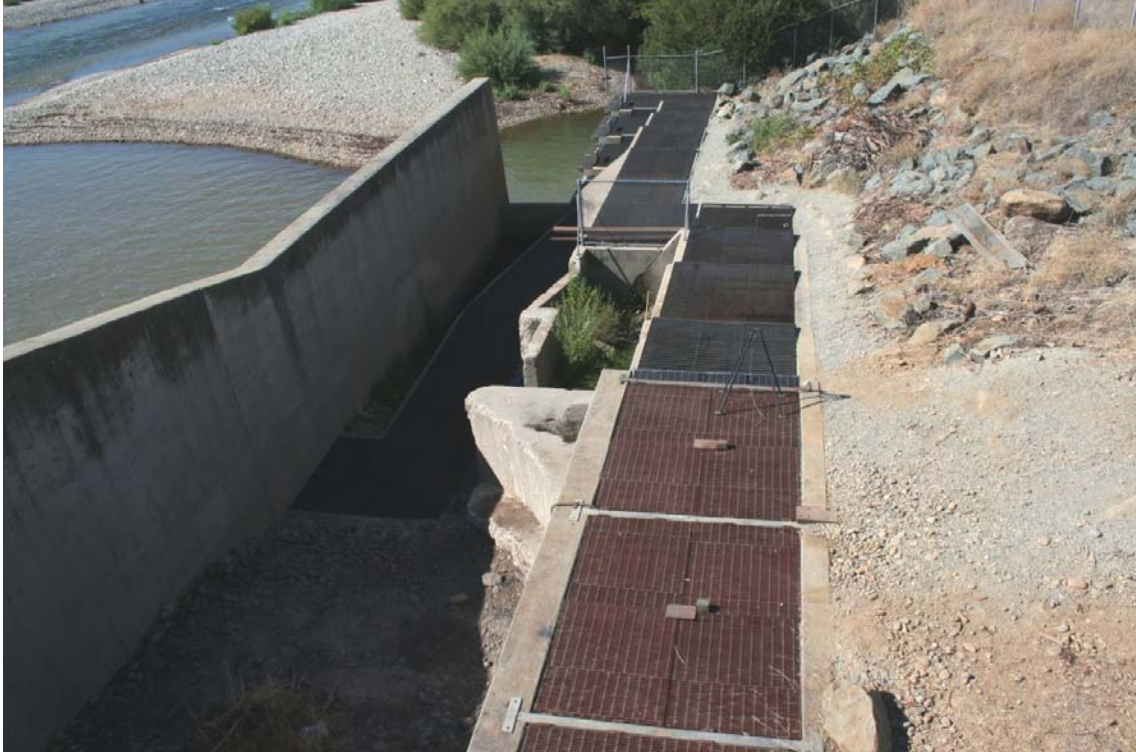
Figure 2-2. North fish ladders at Daguerre Point Dam (Corps 2012c).
