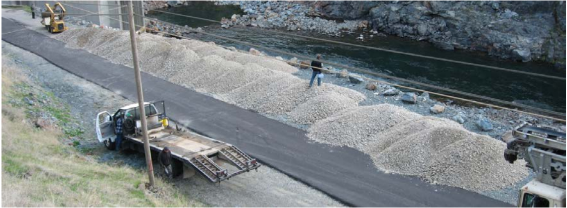
Figure 2.2. 500 short tons of gravel/cobble prior to injection into the Narrows II pool.
