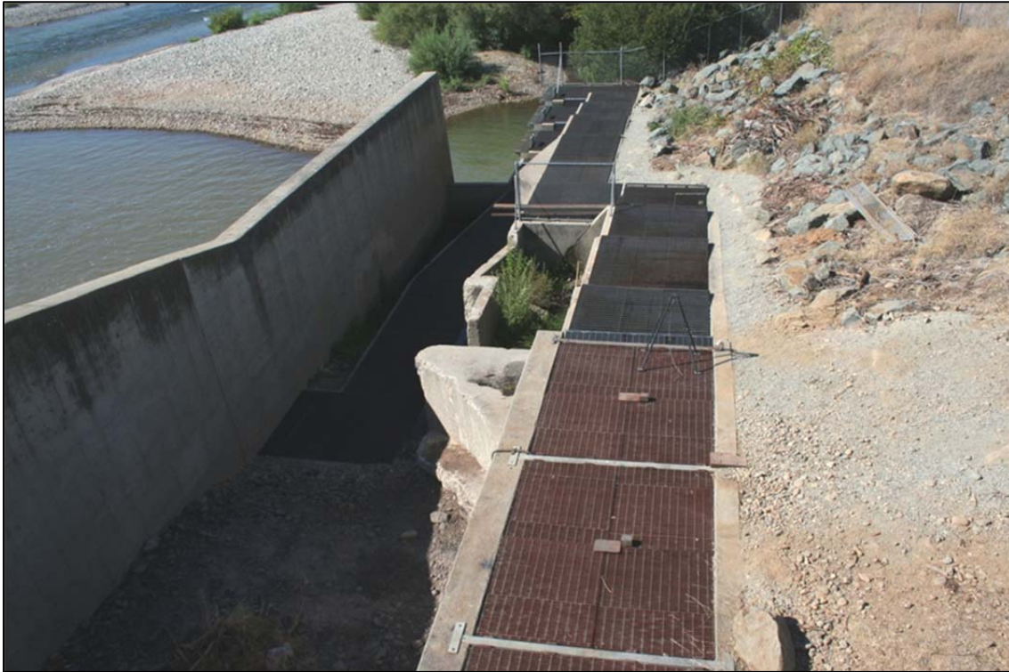
Figure 5-2. North fish ladders at Daguerre Point Dam (Corps 2012c).
