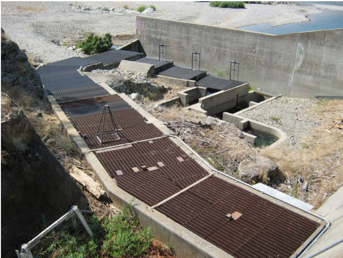
Figure 2-3. South fish ladders at Daguerre Point Dam (Corps 2012c).
