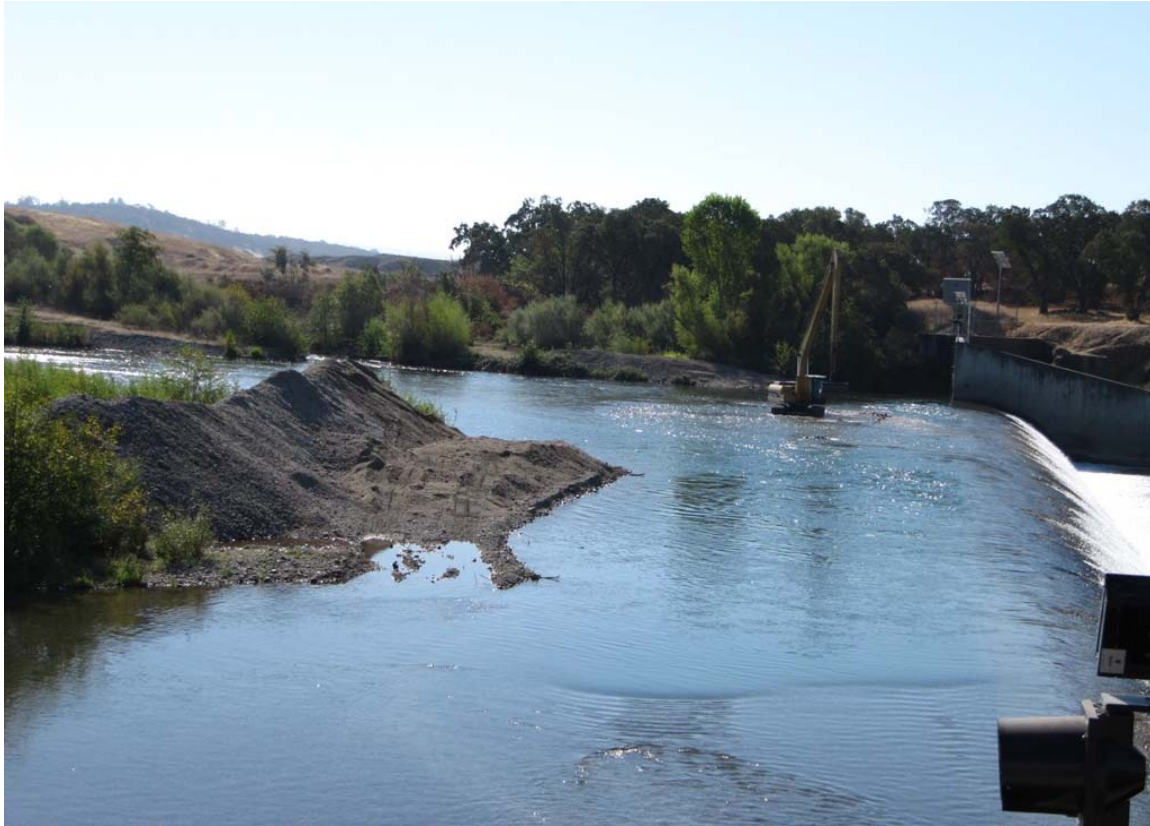
1 2 Figure 2-4. Excavator removing sediment above Daguerre Point Dam during August 2011.
