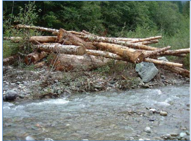
Figure 4. Example of large wood placed on the floodplain will provide low velocity refuge during high flows (Finney Creek in Skagit County, Washington, as shown in Saldi-Caromile et al. 2004).
